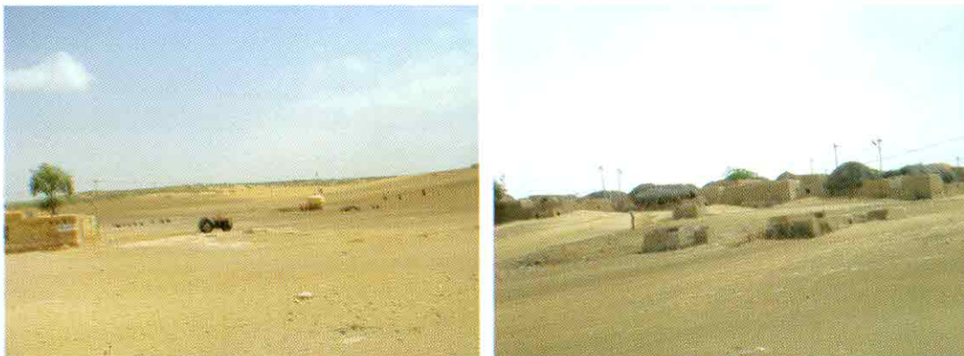
Fig. 8. Scattered rehabilitation with poor conditions
